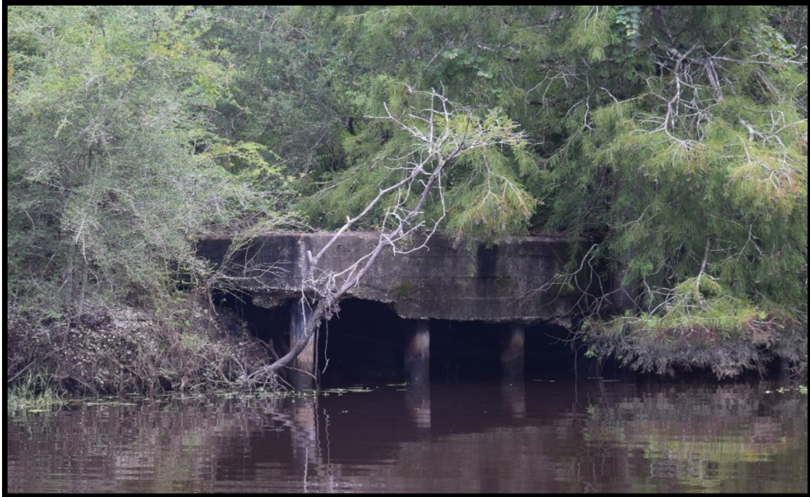
Figure 31: Structure 52-02910 Lacombe Transfer Dock 2
