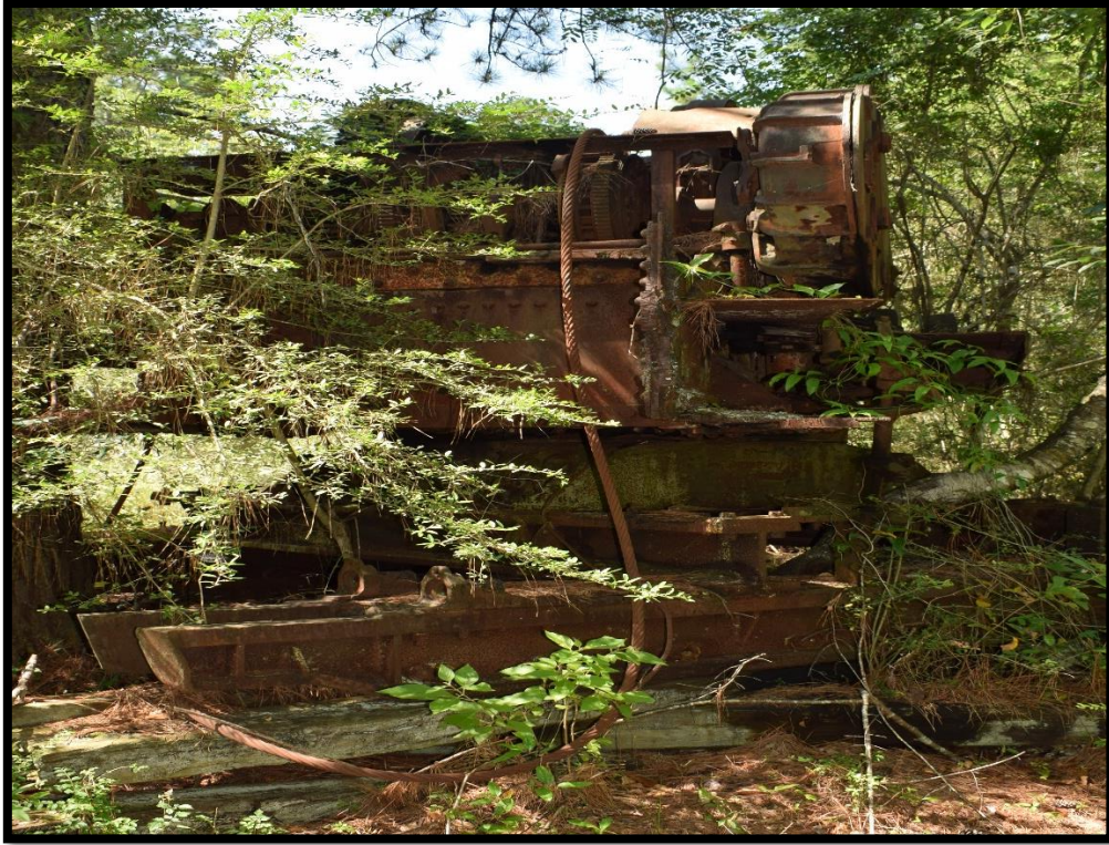
Figure 25: Structure 52-02904 Lacombe Crane
