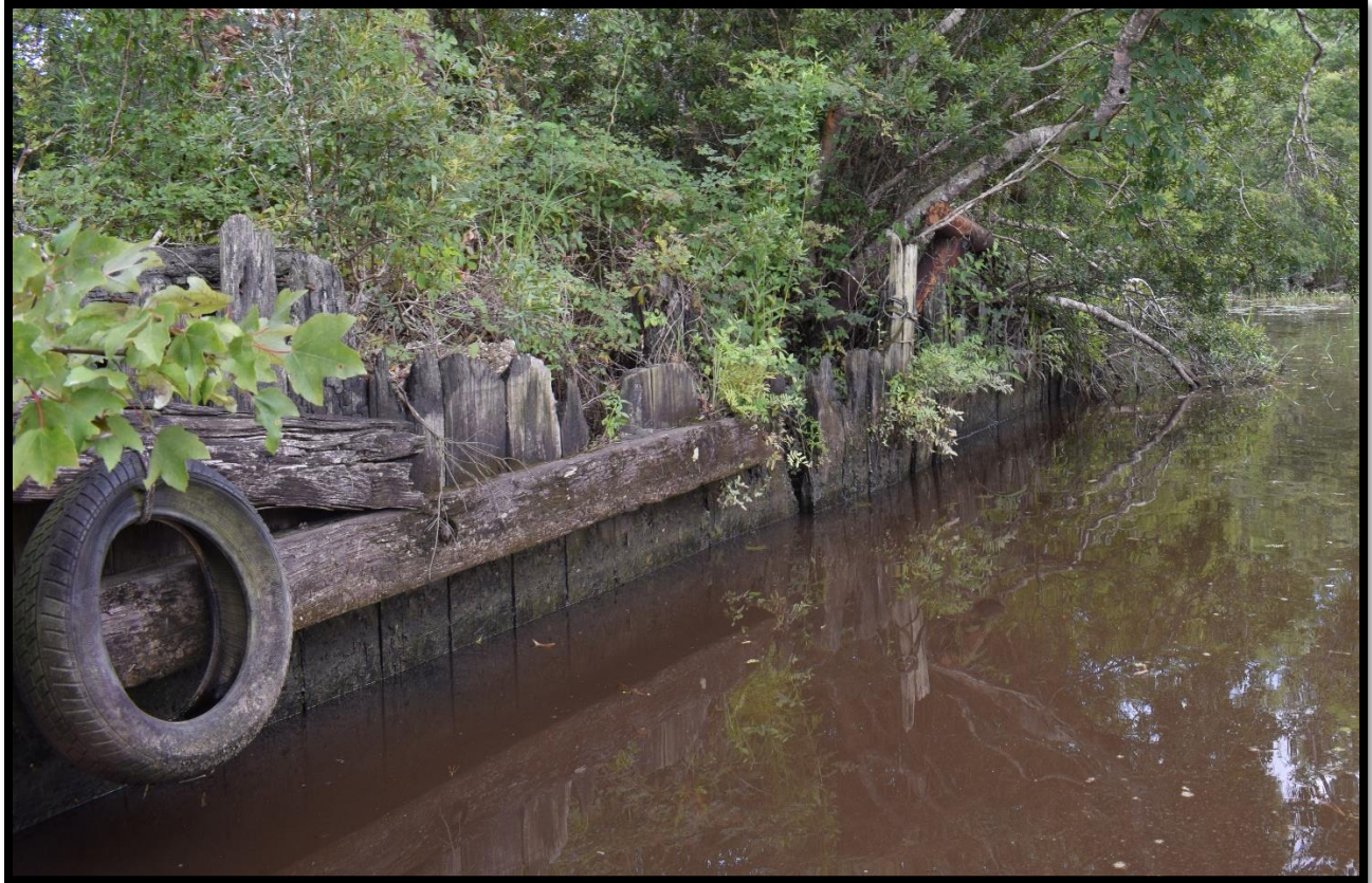
Figure 29: Structure 52-02908 Lacombe Retaining Wall
