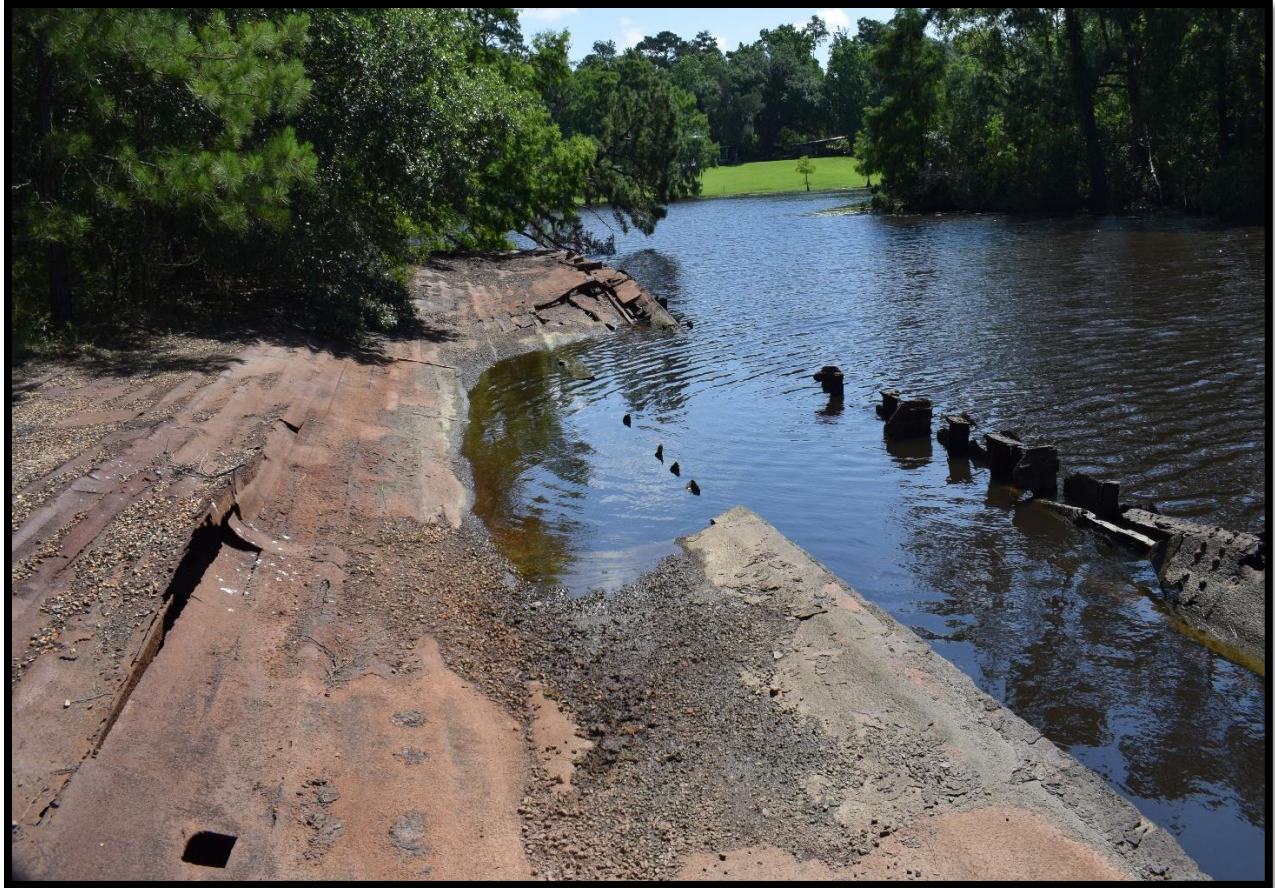
Figure 28: Structure 52-02907 Lacombe Dredge Barge 2
