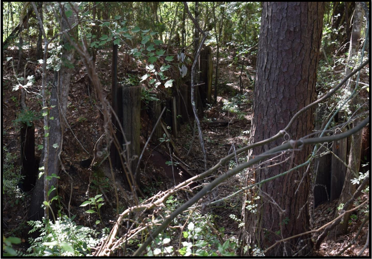
Figure 30: Structure 52-02909 Lacombe Drag Slip
