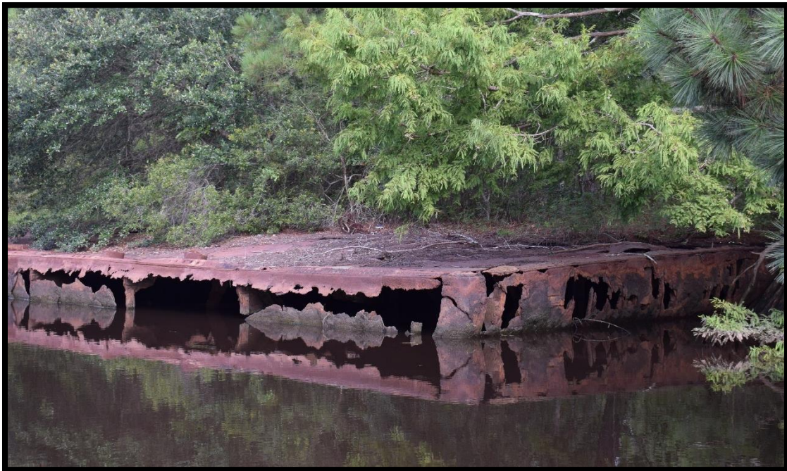
Figure 27: Structure 52-02906 Lacombe Dredge Barge 1
